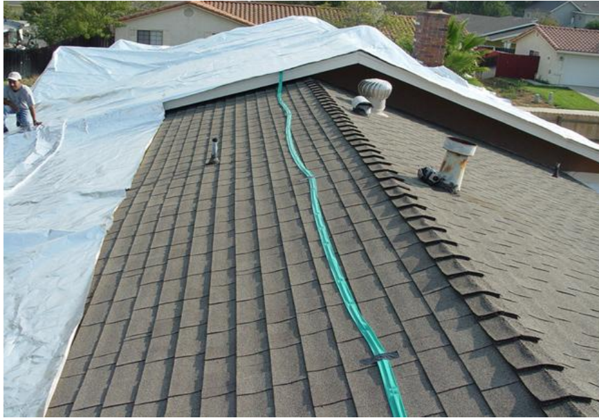
Water Saturation Line Under Fire Shields
